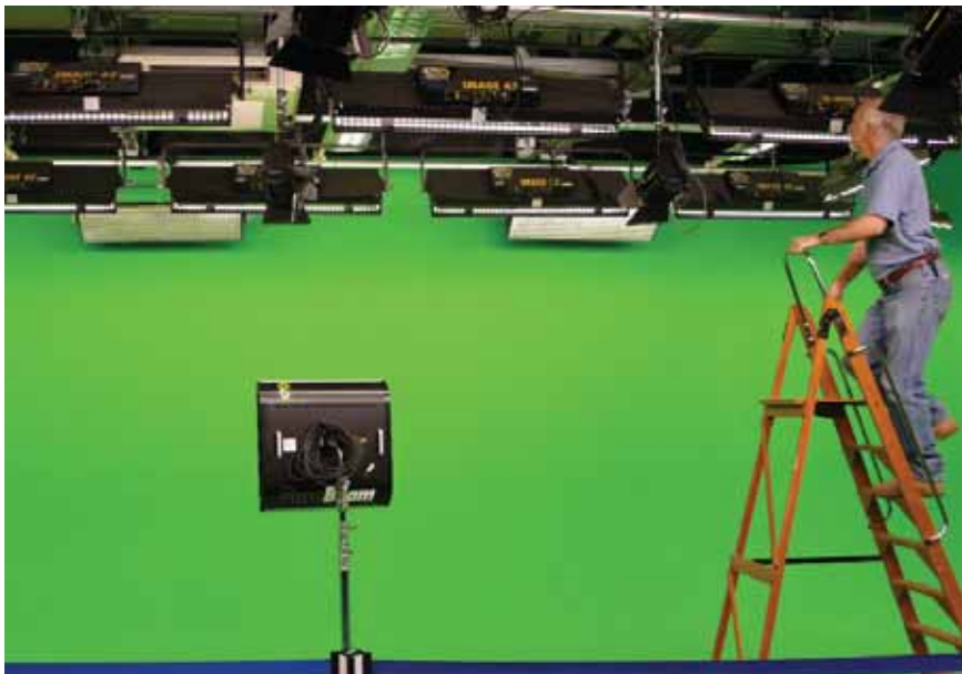
20' x 20' (7m x 7m) visual effects green cyc and floor lighted from above with Kino Flo Image 45 DMX fixtures, lamped with True Match® 3200K full spectrum tubes.
